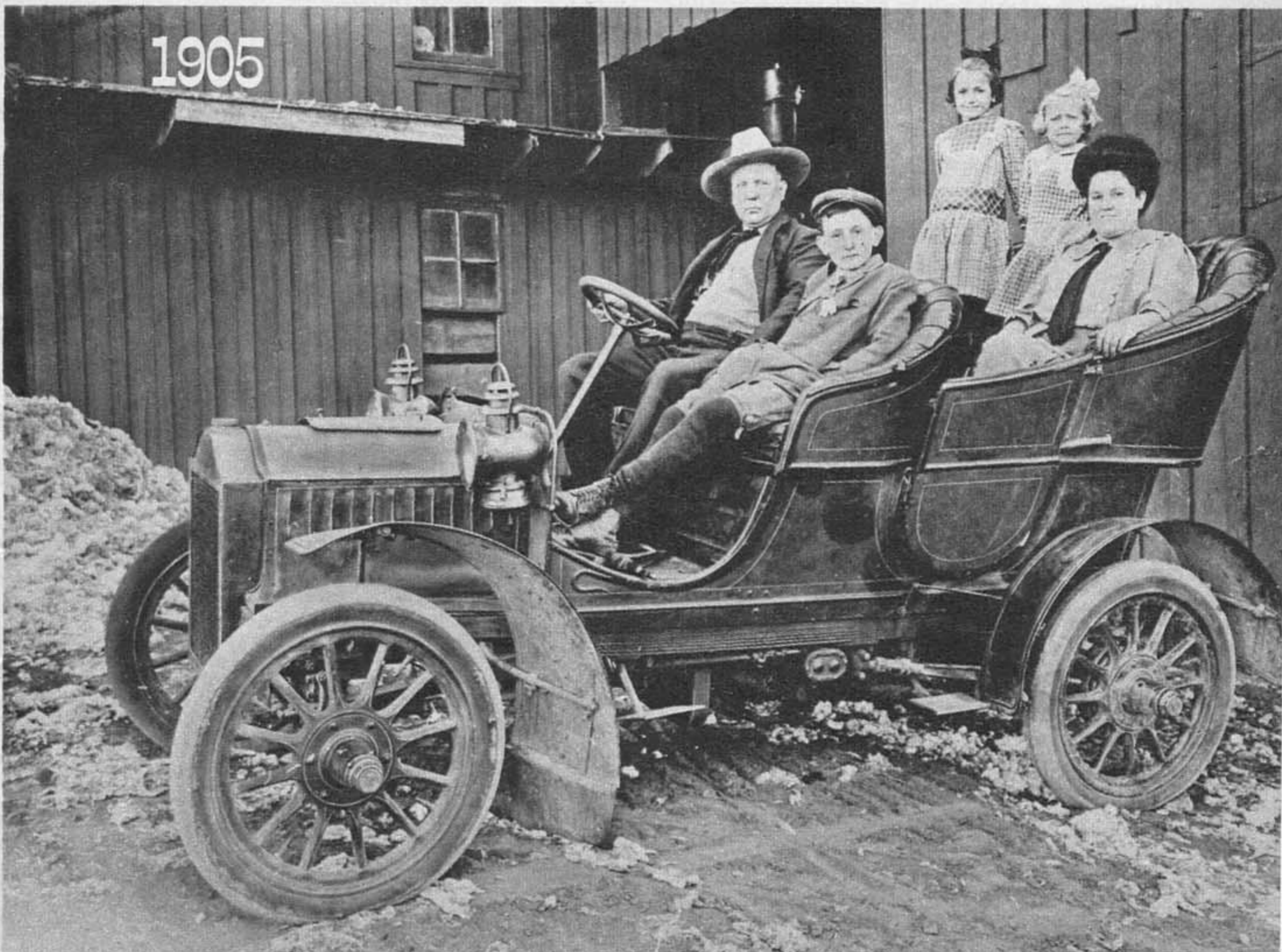
Farmer and family in five-passenger Olds touring car. Powered by a 22 hp two-cylinder, two-stroke engine, it cost $1,400 without top. Featured were flared fenders and long leaf spring. Weight: 2,350 pounds.
